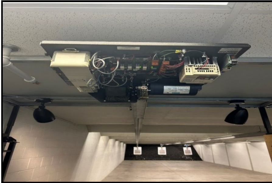
Figure 2. Broken Target Retrieval System Equipment at the Oroville LPOE 10
