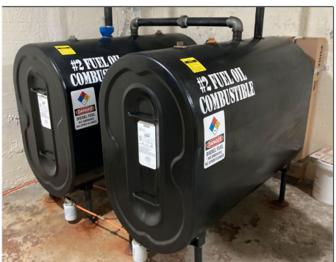
Image 1. Aboveground Fuel Storage Tanks<sup>7</sup>
